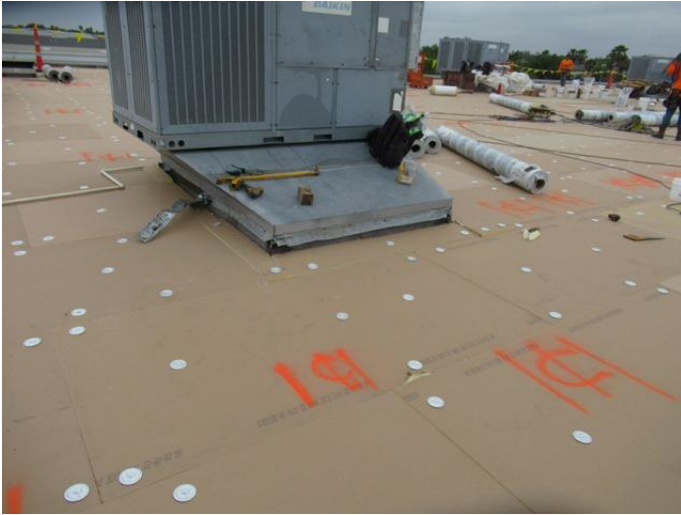
Existing Flashing / Counter Flashing Not Removed Low Flashing Height also Depicted
