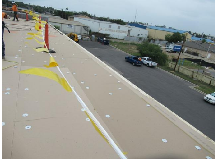
New TPO / Insulation Installation Overview
