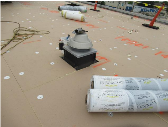
Existing Flashings Not Removed
