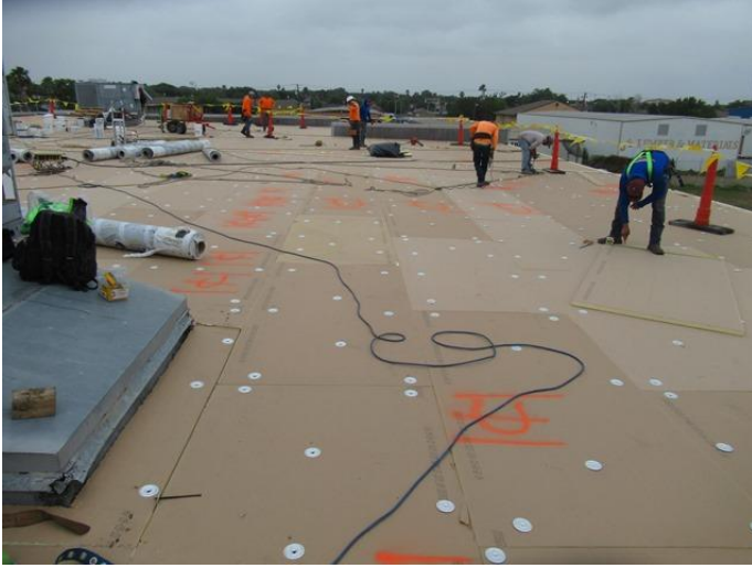
New TPO / Insulation Installation Overview
