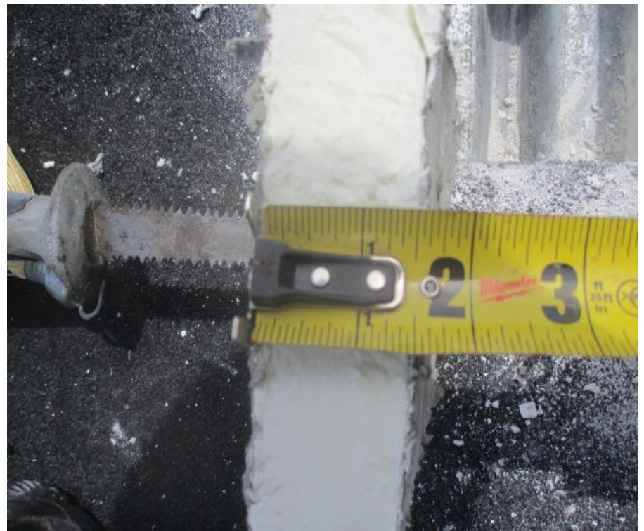
18. Test Cut #5 (Area B): View of roof insulation measurement
