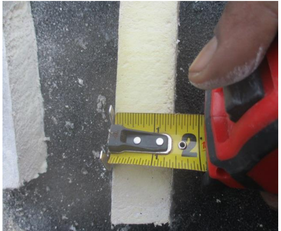
54. Test Cut #6 (Area C): View of roof insulation measurement
