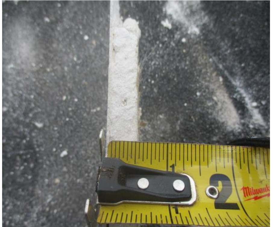
53. Test Cut #6 (Area C): View of DensDeck measurement
