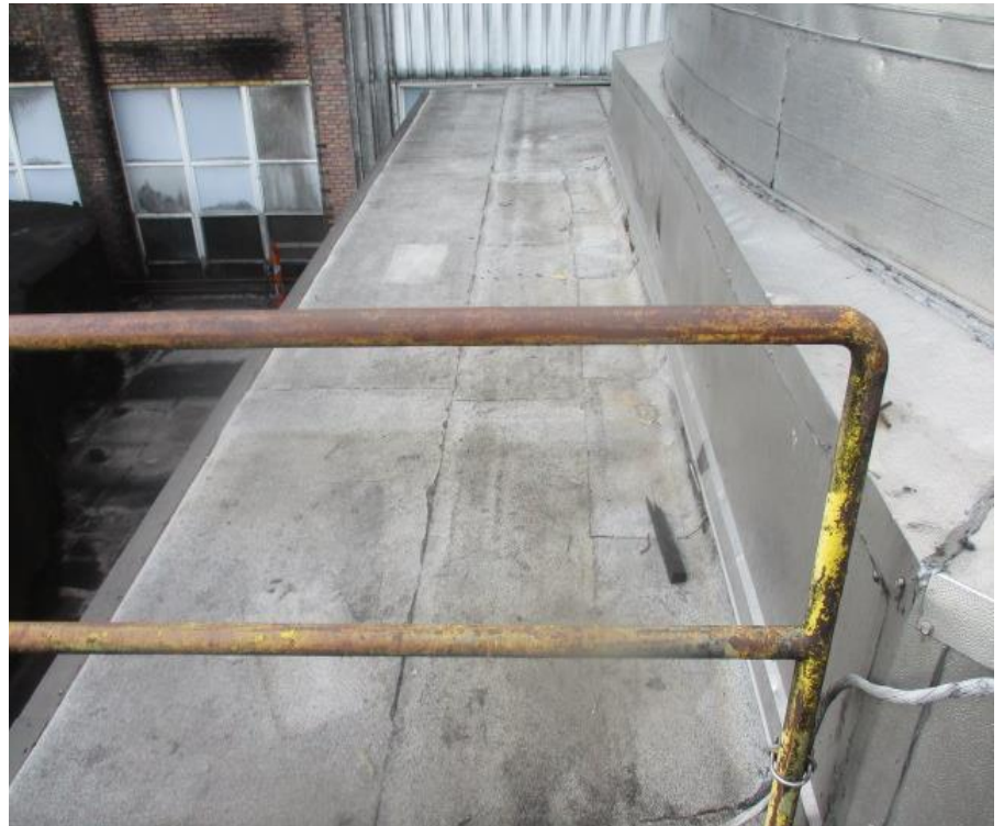
28. Bldg 8 - Area D1 roof system overview
