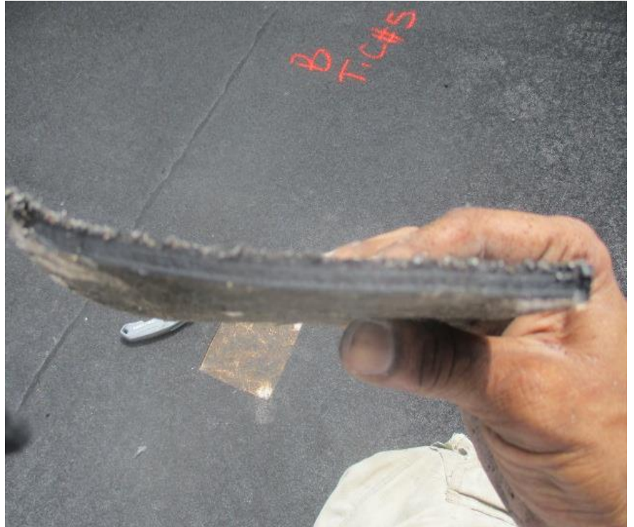
15. Test Cut #5 (Area B): View of modified bitumen plies
