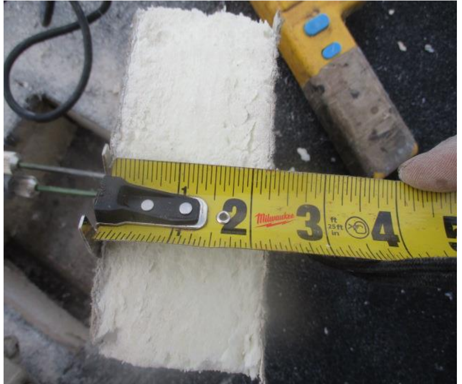
71. Test Cut #12 (Area G): View of roof insulation measurement
