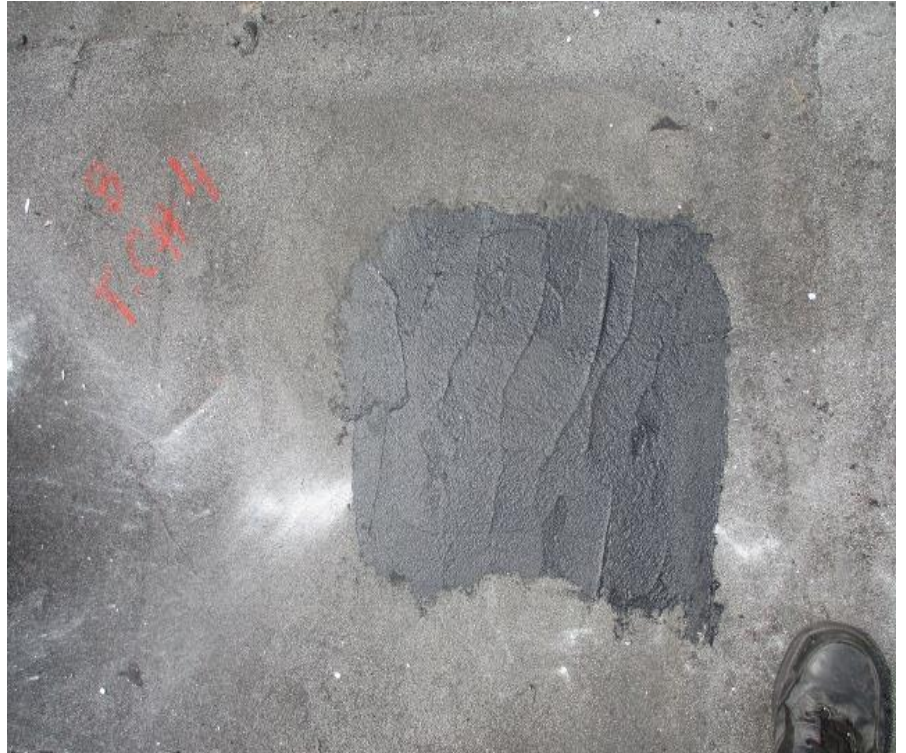
23. Test Cut #4 (Area B1): View of RCS repair
