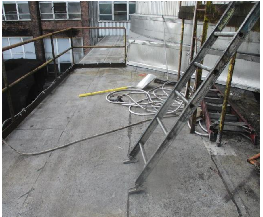
32. Bldg 8 - Area D1 roof system overview
