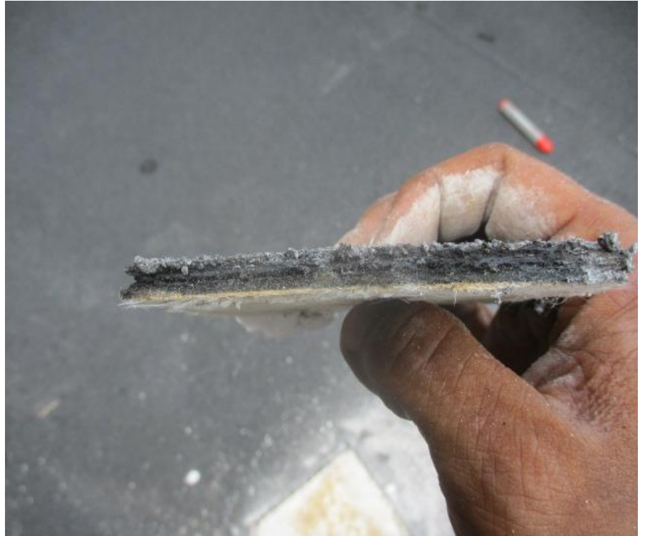
51. Test Cut #6 (Area C): Modified bitumen plies
