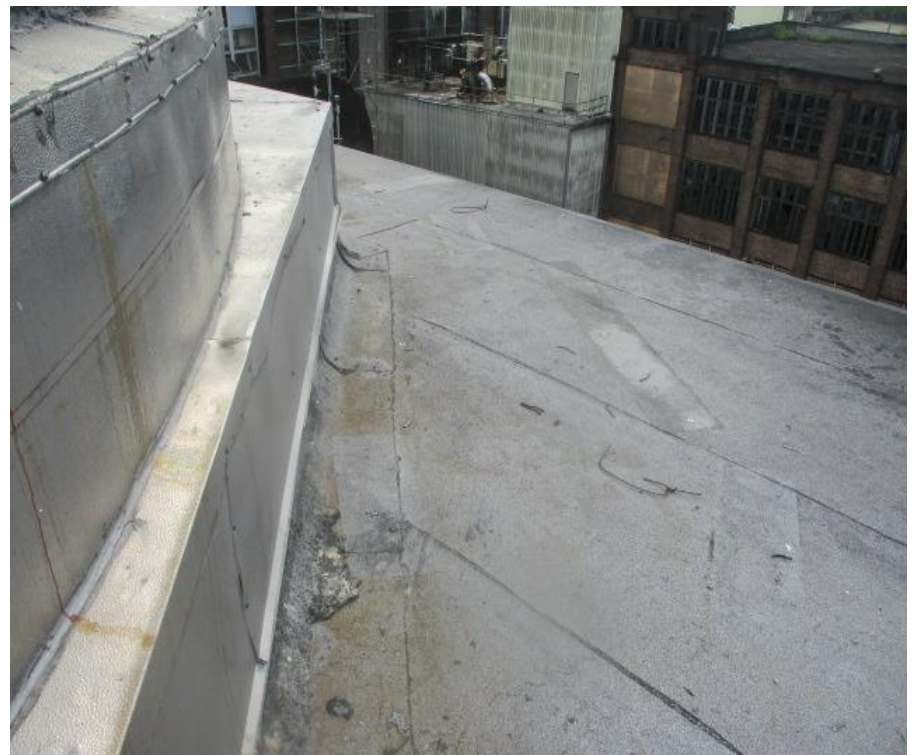
46. Bldg 8 - Area E2 roof system overview
