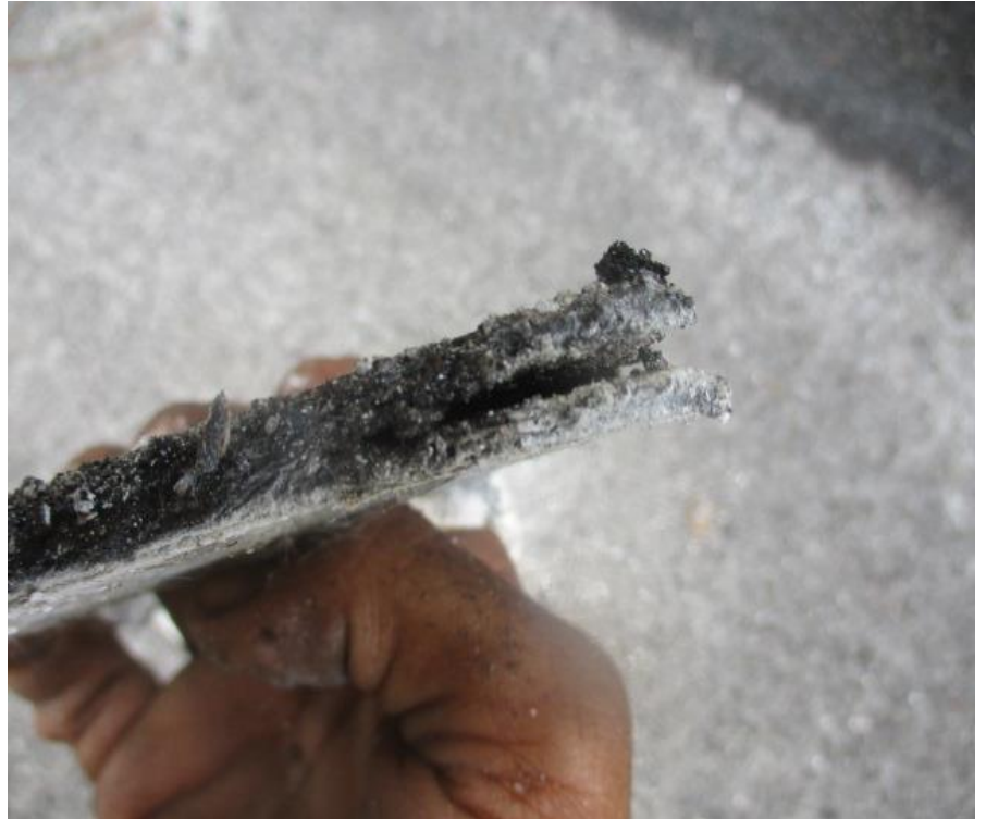
57. Test Cut #9 (Area F): Modified bitumen plies
