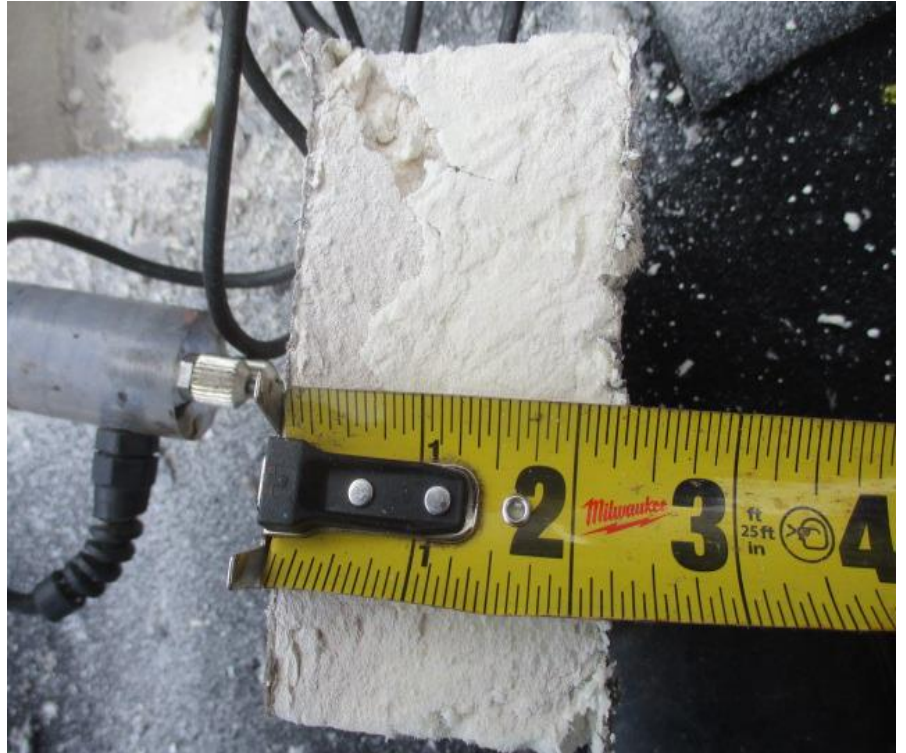
49. Test Cut #1 (Area A): View of roof insulation measurement
