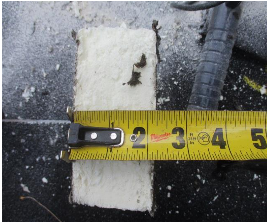
50. Test Cut #1 (Area A): View of roof insulation measurement
