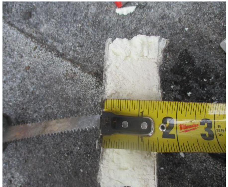
60. Test Cut #9 (Area F): View of roof insulation measurement
