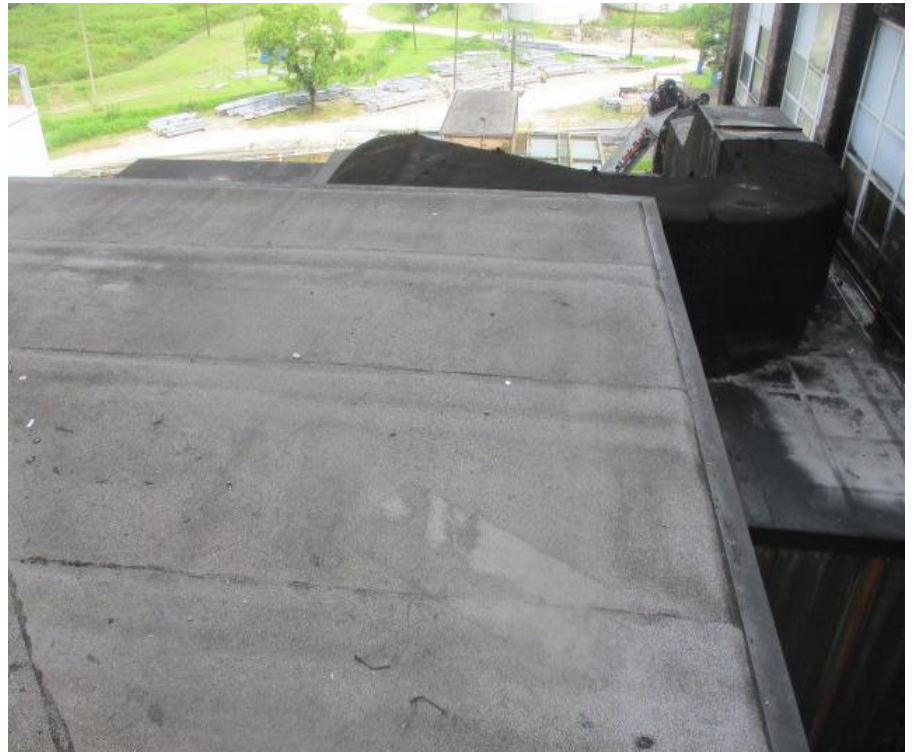
26. Bldg 8 - Area D1 roof system overview
