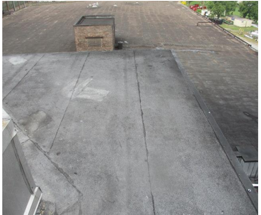
34. Bldg 8 - Area D1 roof system overview
