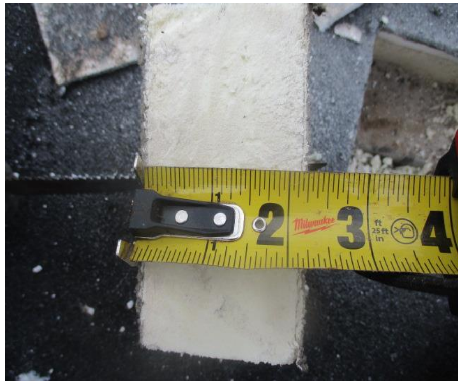
66. Test Cut #11 (Area G): View of roof insulation measurement
