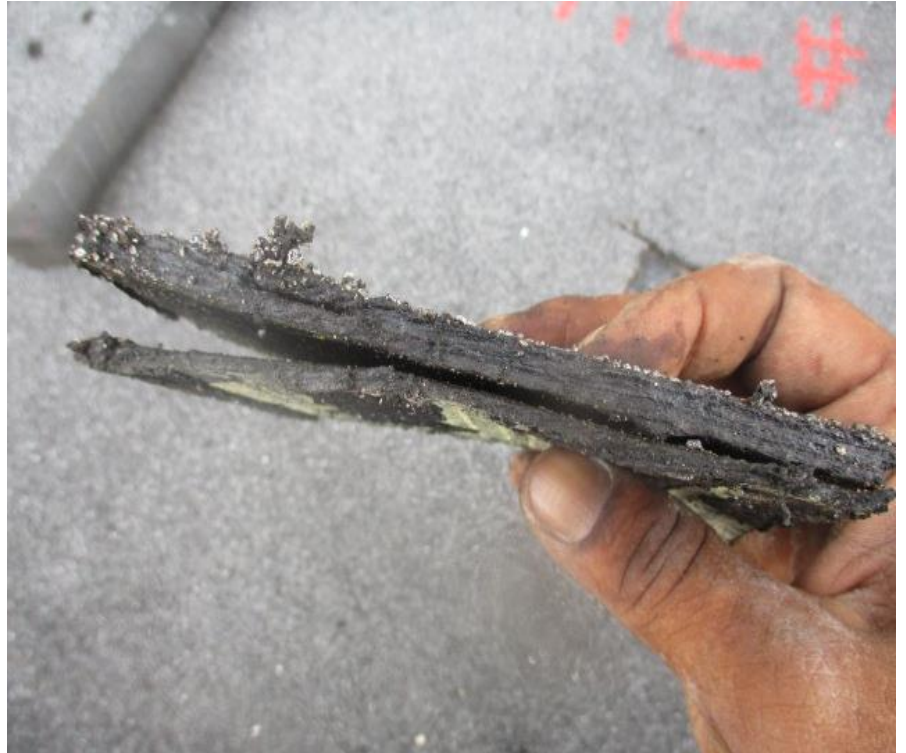
21. Test Cut #14 (Area I): View of modified bitumen plies
