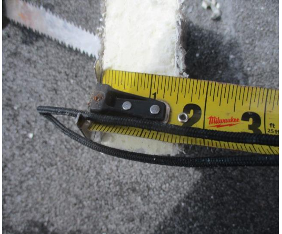
21. Test Cut #4 (Area B1): View of roof insulation measurement
