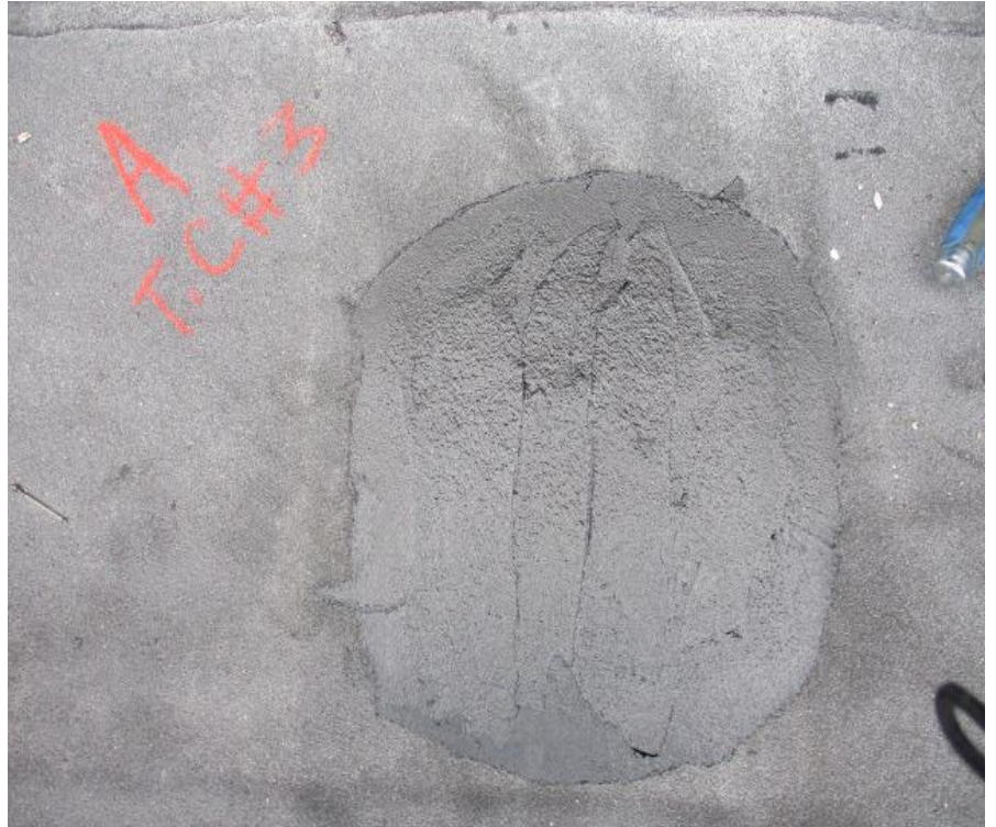
59. Test Cut #3 (Area A): View of RCS repair
