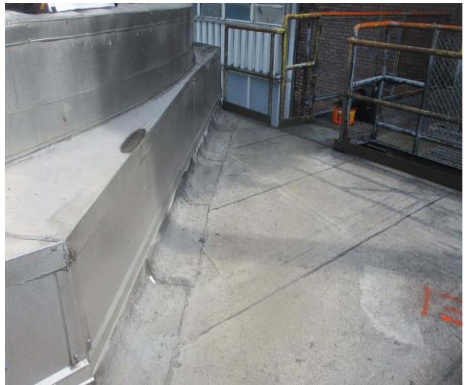
50. Bldg 8 - Area E2 roof system overview
