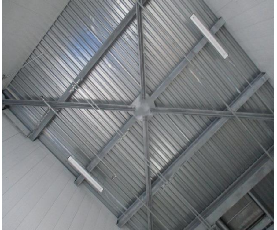
5. View of underside of roof deck at building interior
