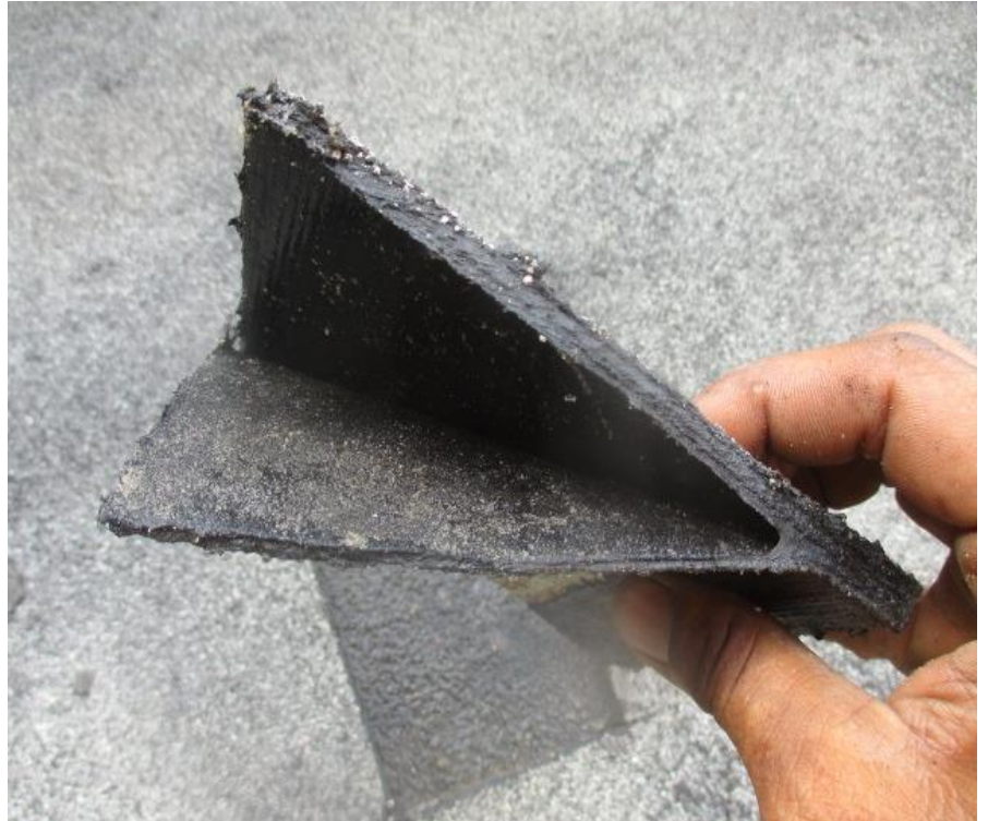
73. Test Cut #10 (Area E2): View of modified bitumen plies
