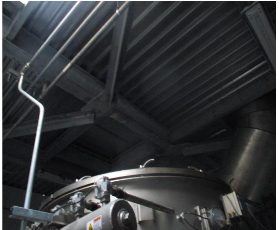
6. View of underside of roof deck at building interior
