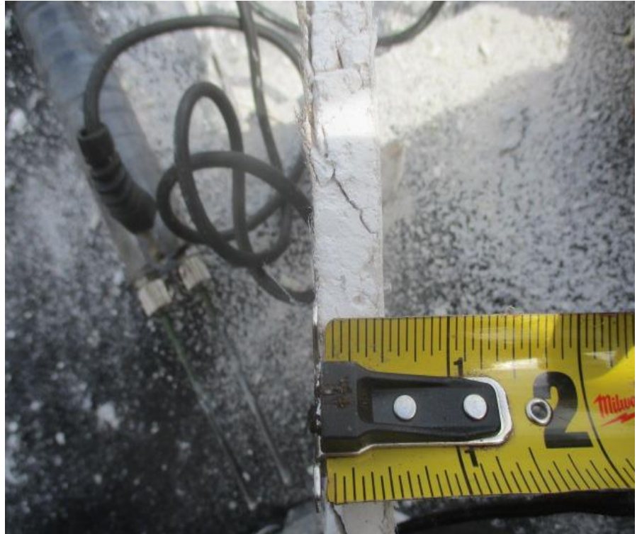
17. Test Cut #5 (Area B): View of DensDeck measurement
