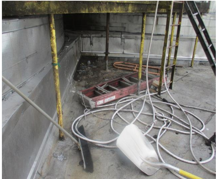
30. Bldg 8 - Area D1 roof system overview
