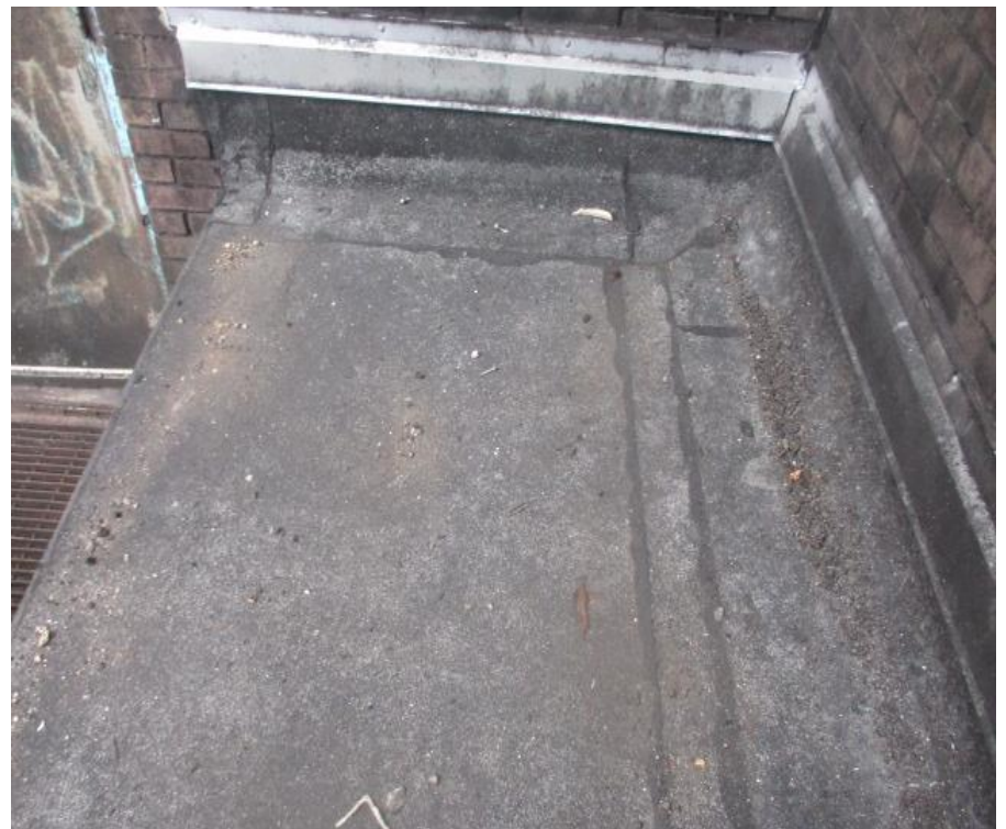
10. Bldg 8 - Area E1 roof system overview
