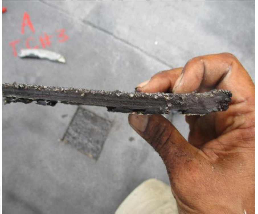
57. Test Cut #3 (Area A): View of modified bitumen plies
