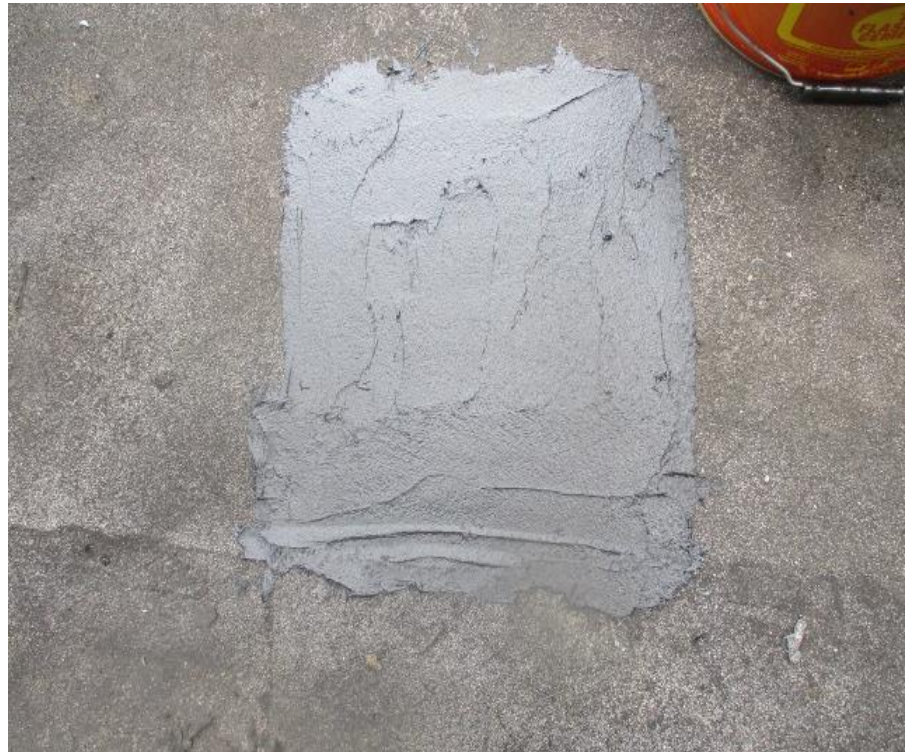
72. Test Cut #7 (Area D): View of RCS repair
