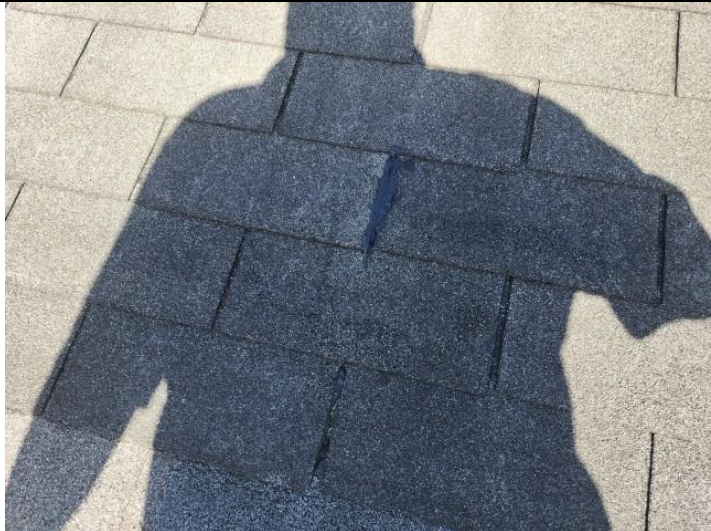
Repaired Shingles on Bldg 1
