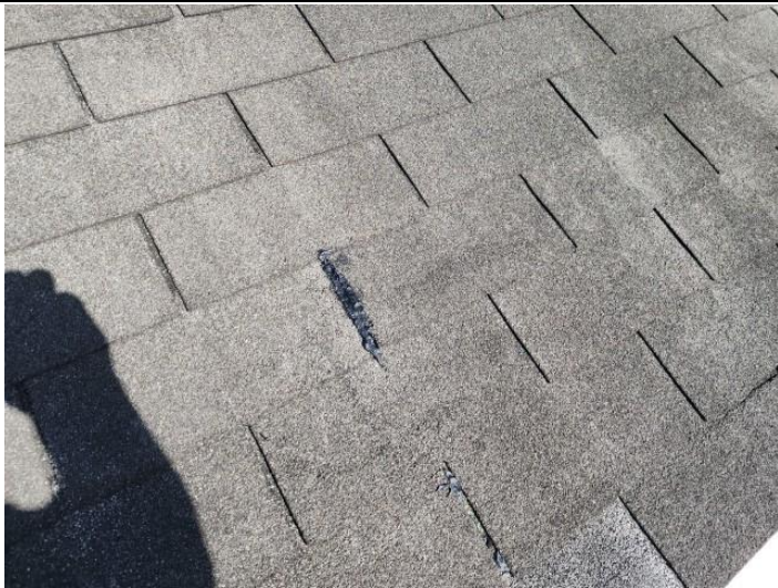
Repaired Shingles on Bldg 1
