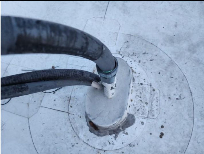
Open condition at conduit
