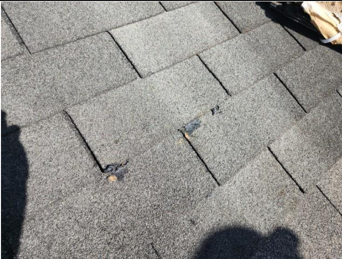
Repaired Shingles on Bldg 1
