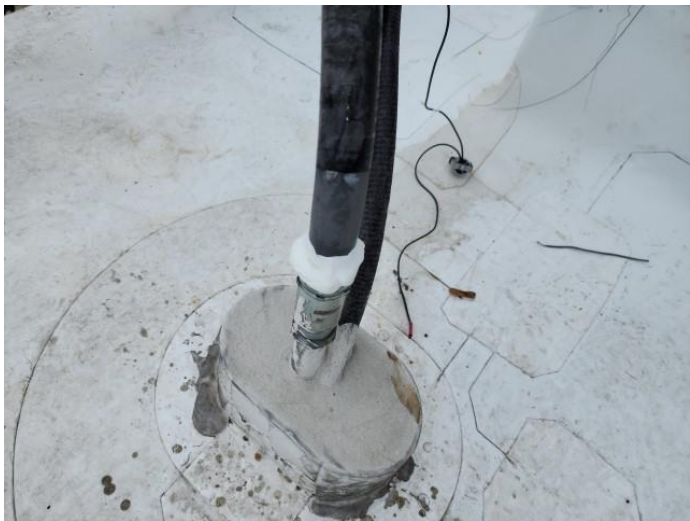
Open condition at conduit – Repair made with sealant
