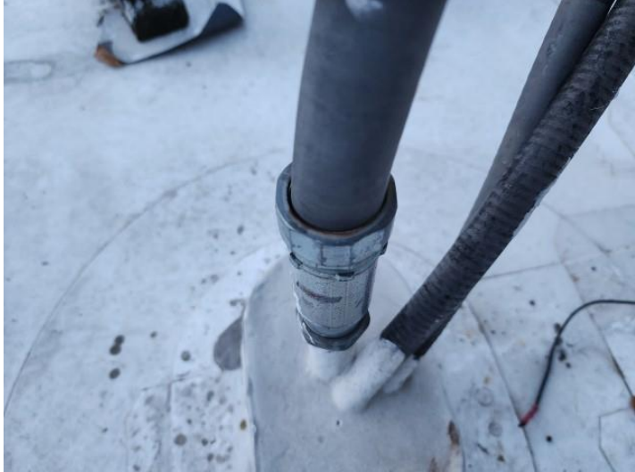
Open condition at conduit
