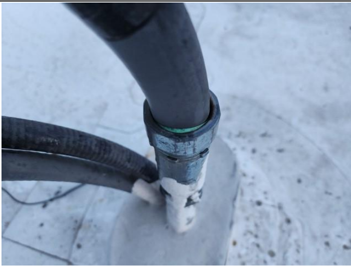
Open condition at conduit
