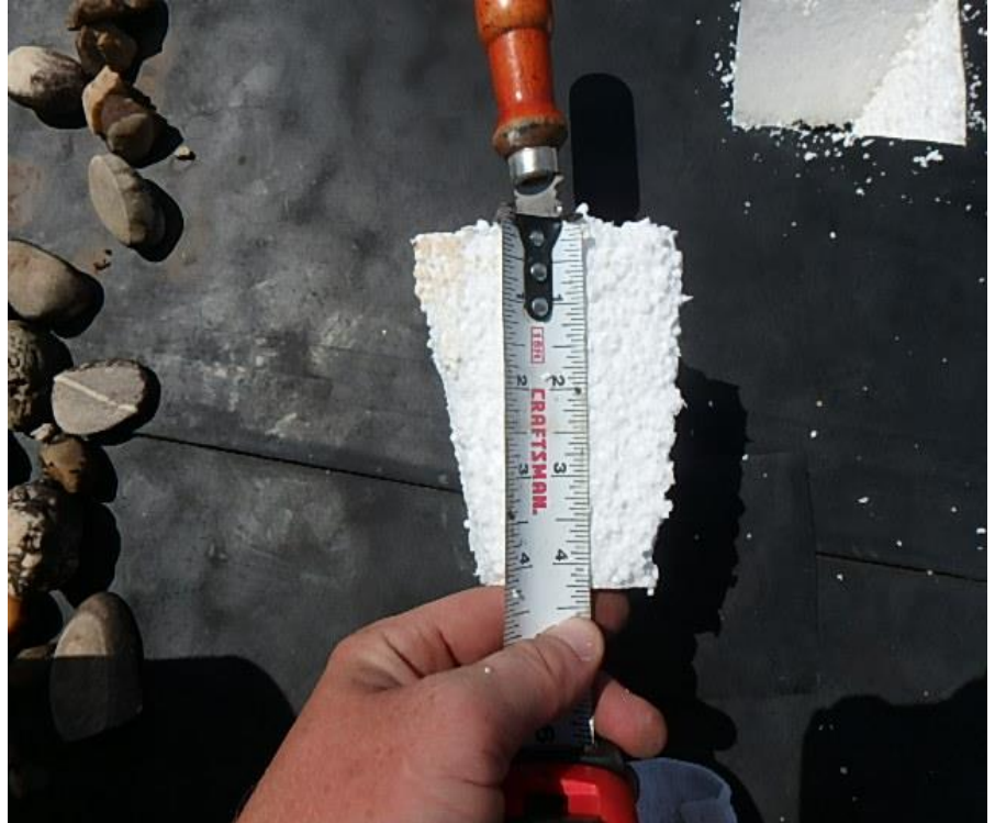
67. View of roof insulation measurement on Bldg 1 - Area C
