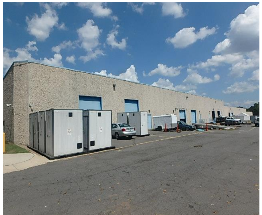
6. Building exterior rear elevation overview
