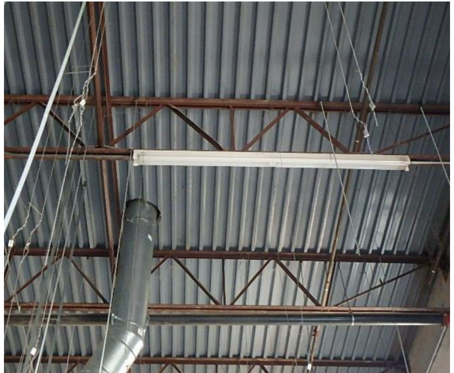
10. View of underside of roof deck at building interior
