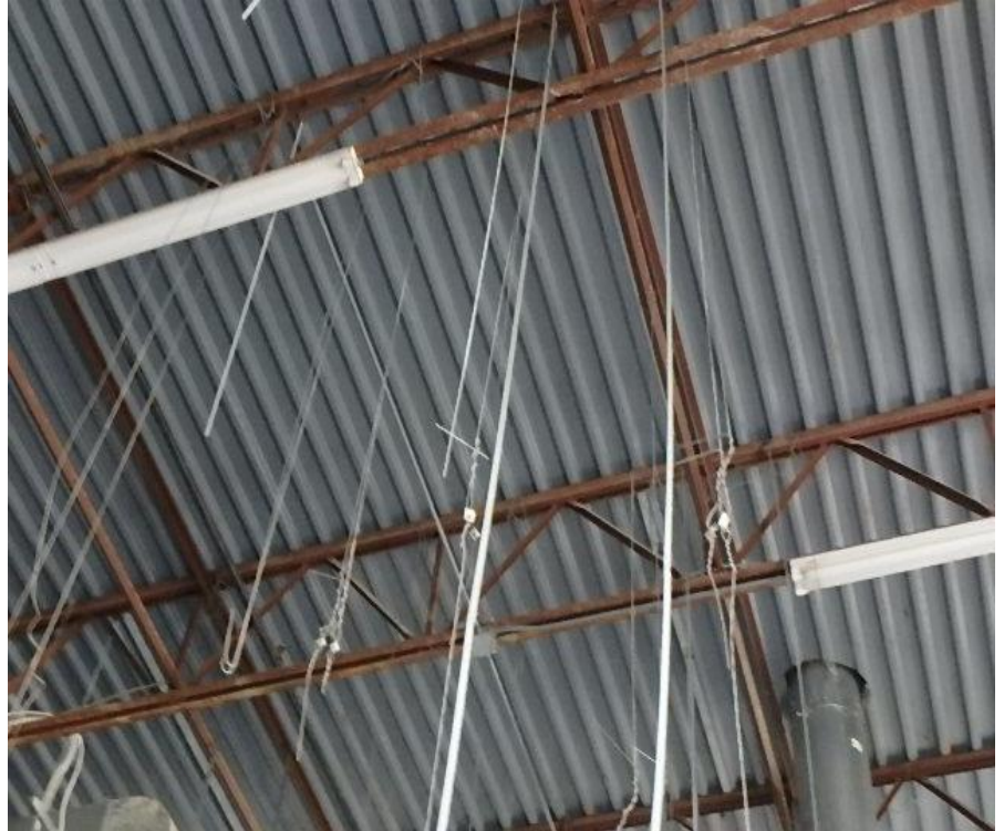
9. View of underside of roof deck at building interior
