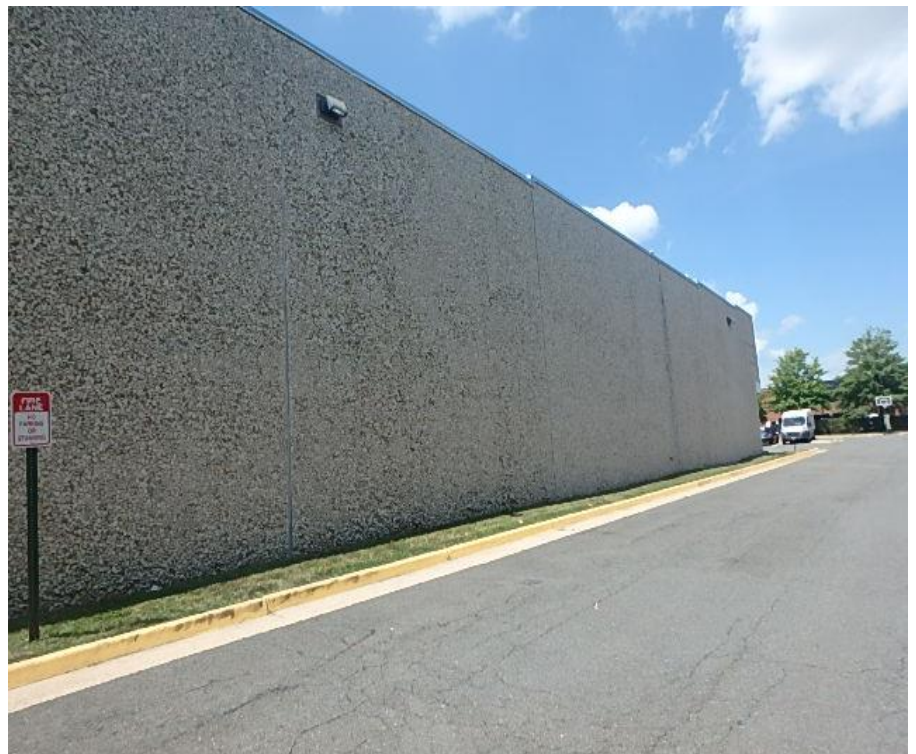
8. Building exterior side elevation overview
