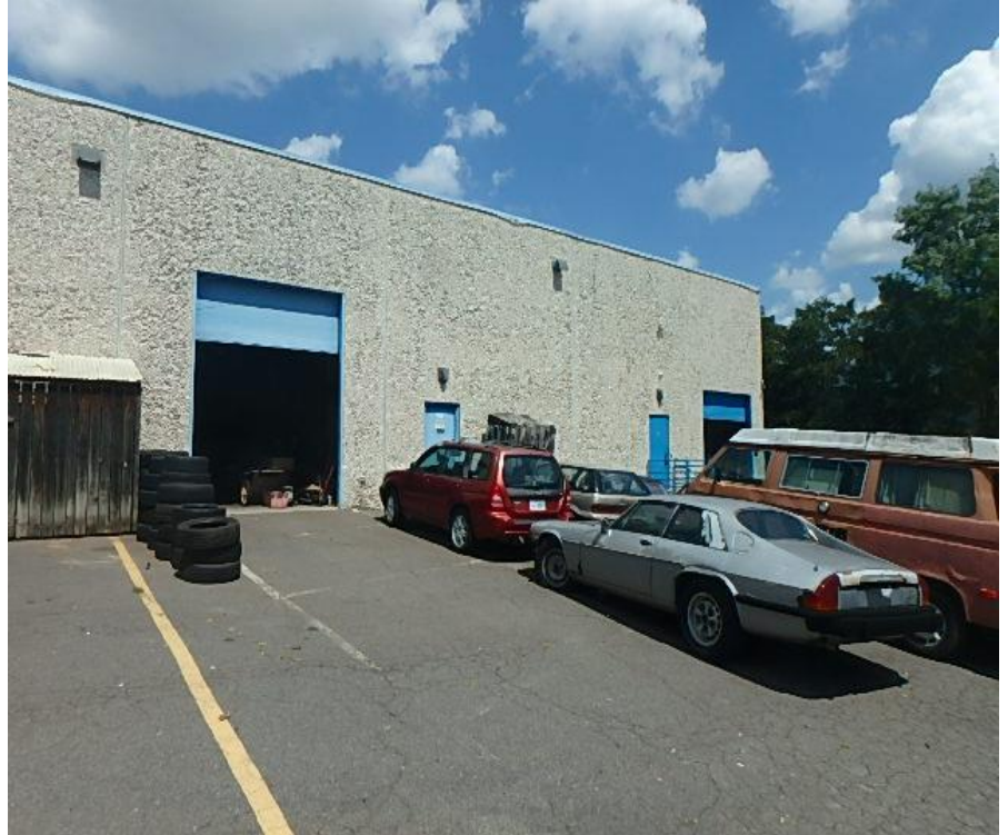
7. Building exterior rear elevation overview
