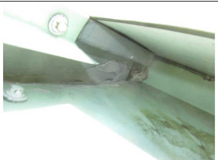
Close up view identifying the poor detailing at the roof panel / ridge cap / rake edge
